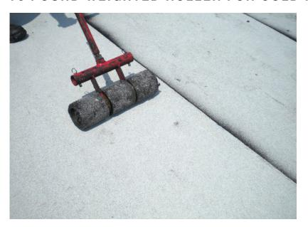
Tremco requires all cold applied POWERply top membranes to be fully rolled into the adhesive immediately after application. A weighted roller improves the contact of the back of the POWERply membrane with the adhesives, to minimize the potential for voids within the roof membrane system.
