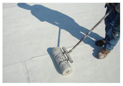
POWERply T24 is a SBS modified bitumen membrane with a factory applied a white acrylic coated surfacing.
