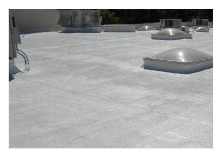
If touch-up is required on the POWERply T24, Solargard 6083 is recommended. No special surface prep is required, except that surface must be clean and dry.
